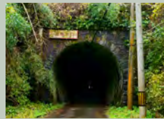
10 Sorojidani Tunnel (401 m)
