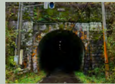
12 Habara Tunnel (979 m)
