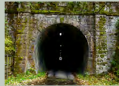
5 Ashitani Tunnel (223 m)
