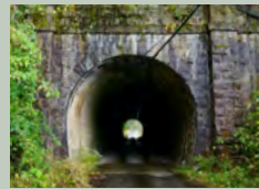
11 Funagaya Tunnel (64 m)
