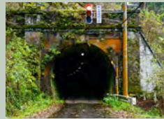
4 Iradani Tunnel (467 m)
