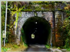
8 No. 1 Kannonji Tunnel (82 m)
