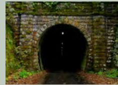
7 No. 2 Kannonji Tunnel (310 m)
