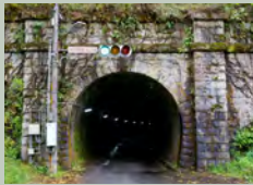
1 Yunoo Tunnel (368 m)
