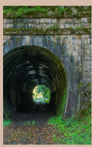
Kotone Tunnel (56m)
