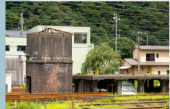
Imajo Station's old water tower and coal supply platform, which were used to refuel steam locomotives, can still be seen at the station, for a unique contrast to today's railroad.
